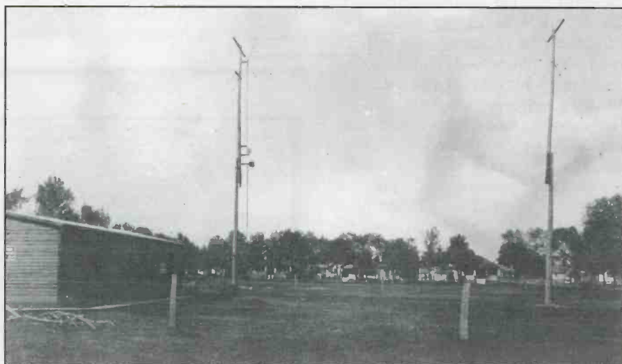
The original KFKX antenna system and transmitter building. It was located in the city park in Hastings. (Photo courtesy Broadcast Pro-File)
